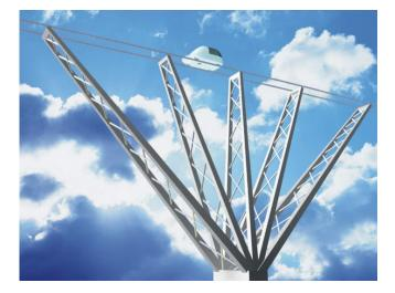
Fig. 22. Supporting mast of great height combined with a vertical curve
