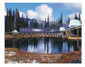
Fig. 21. Anchor support combined with a station and track curve
