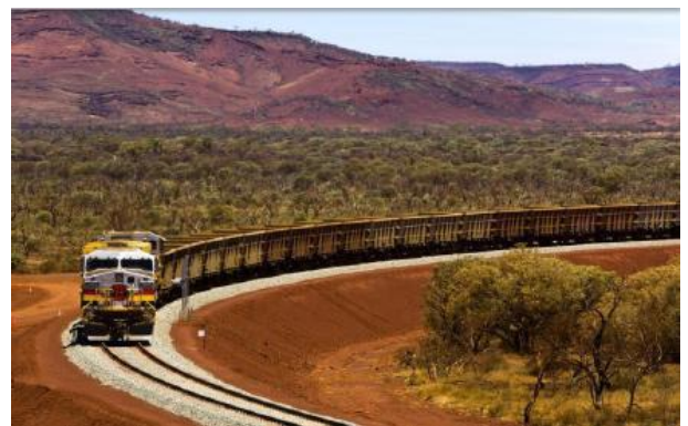
Heavy Haul Train, Very High Embankment, High Volume Earthworks, Large Footprint
