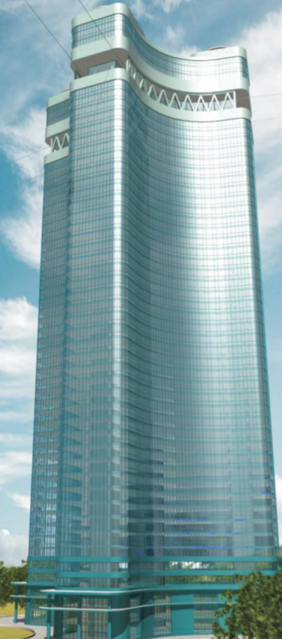
Appearance of YTS high-rise buildings-stations
