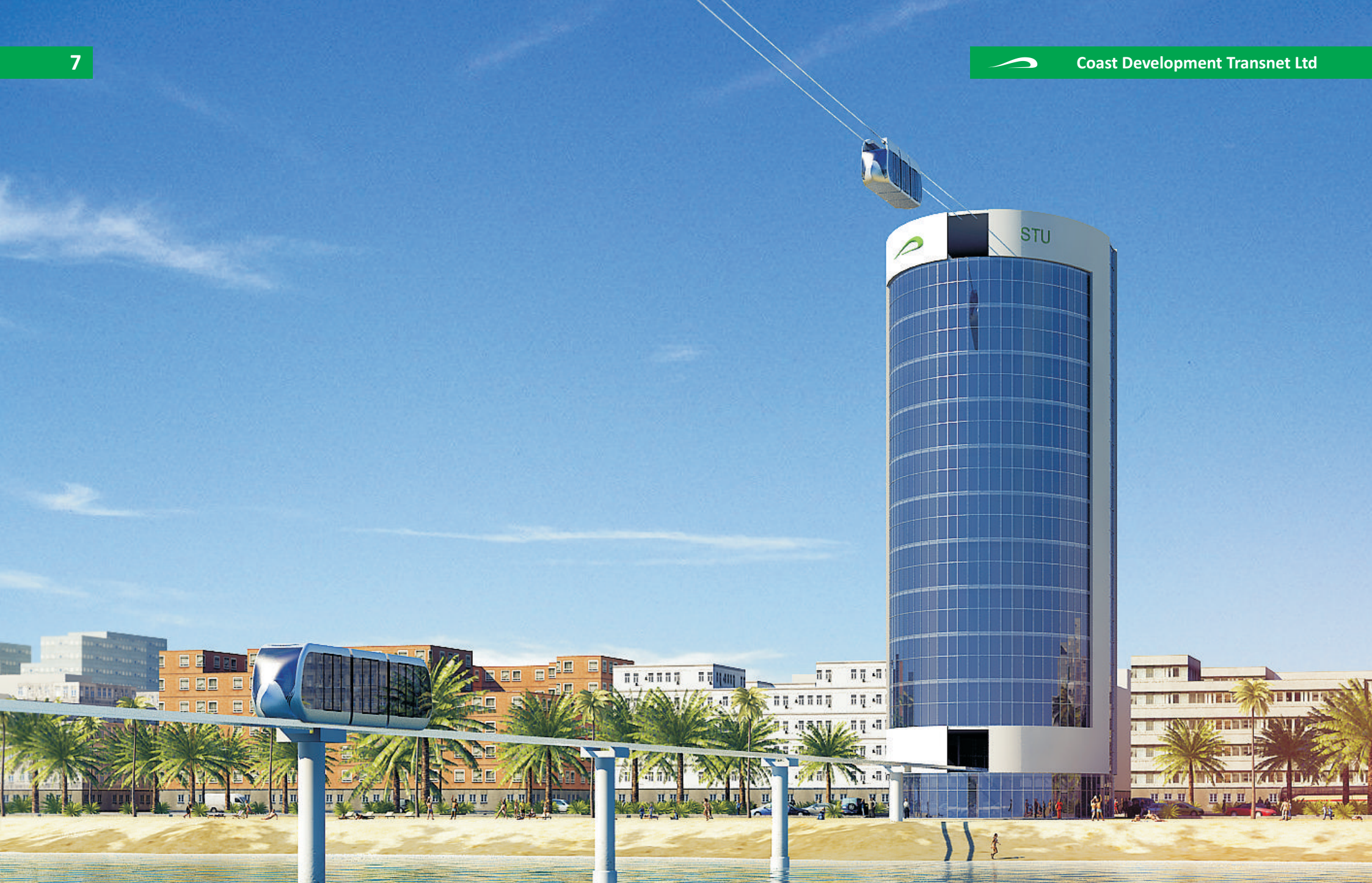
Multi-functional building with “second level” and “third level” YTS station
