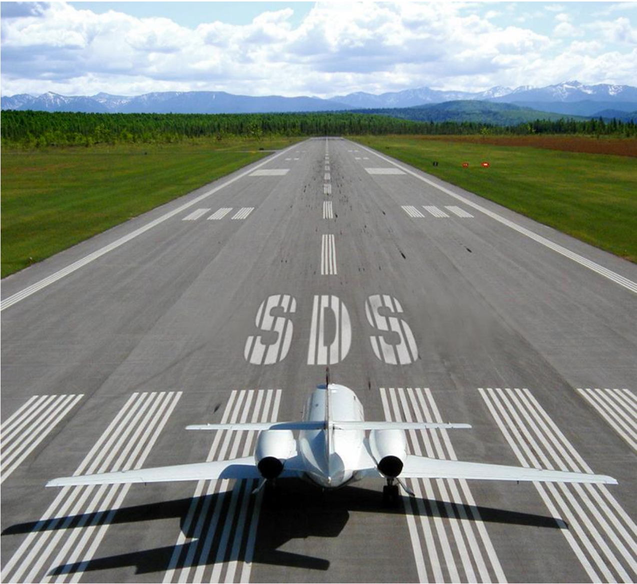
Fig. 11. String runway built without compensation joints (longitudinal and lateral)
