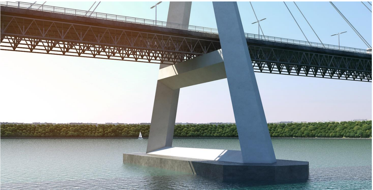
Fig. 10. Side view of the longitudinal sting trusses supporting the cable bridge road
