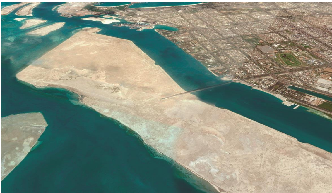
Bird's eye view of Al Hudayriat Island (Google Earth), 2015.
