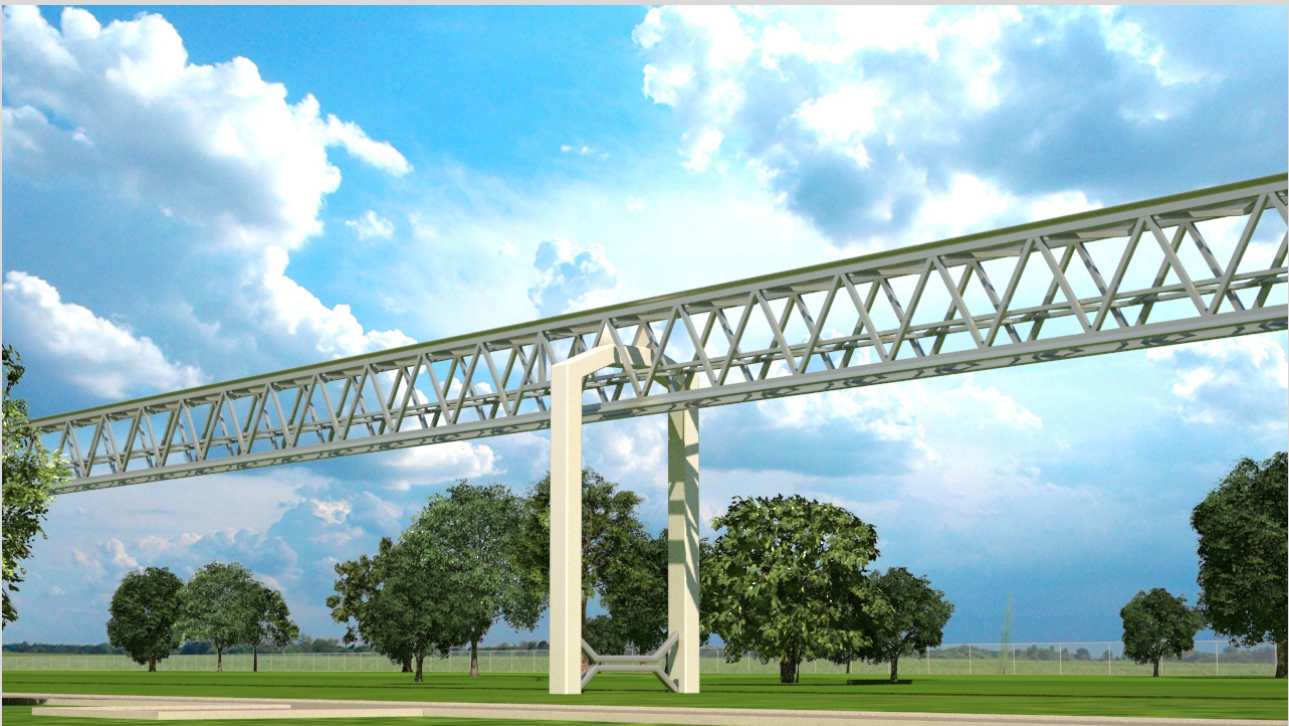
Figure 3.9 – Example of string-trussed track structure
